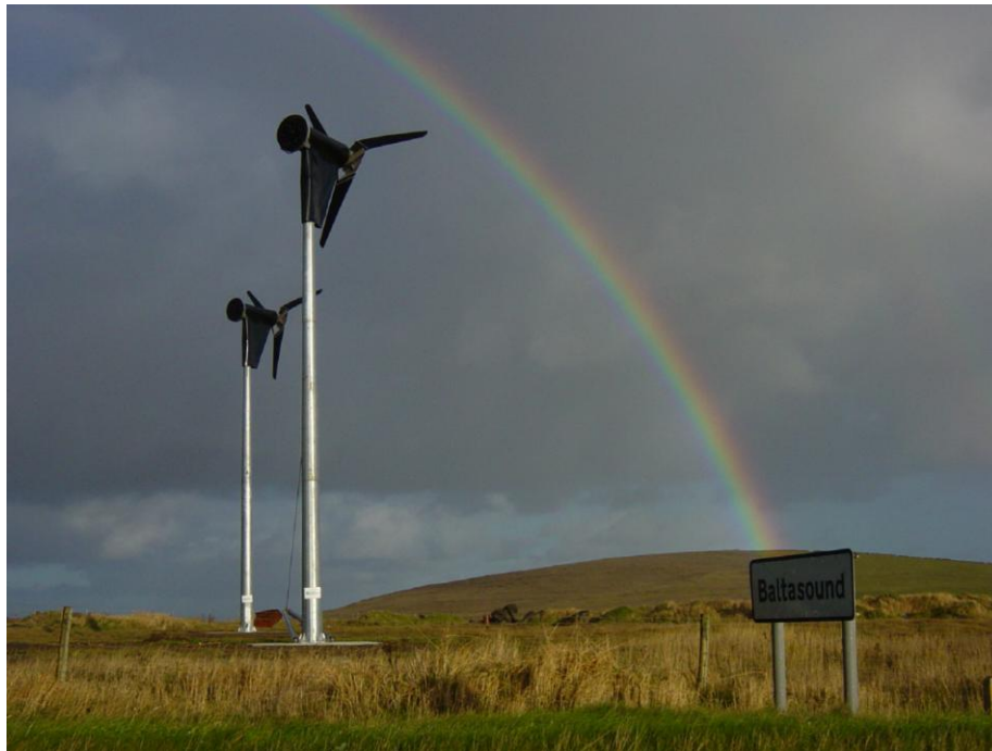
Figure 3: The two wind turbines that provide the primary power source for PURE
